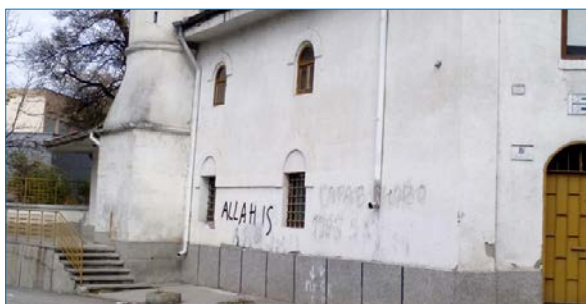
Figure 8: Graffiti on the Plevna Mosque. The insults have since been covered.
